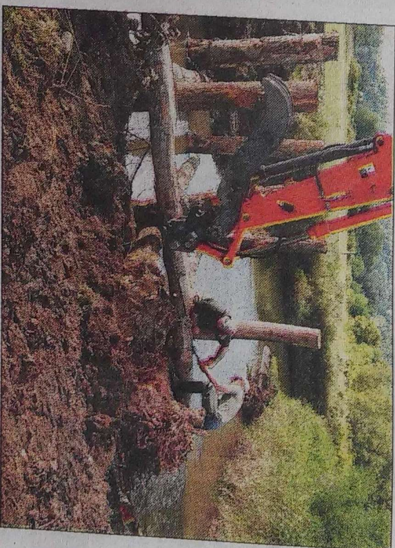
Workers from Riverlogic Solutions of Wellsville, Pa., install logs as part of the trout habitat restoration project on Salmon Creek at a site off Farnum Road in Salisbury.
